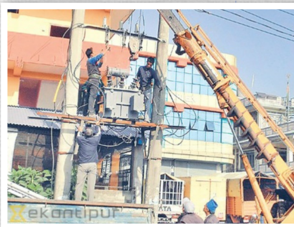
Removing a wrecked transformer
